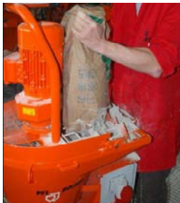
Fig. 32: Fill in bagged material
