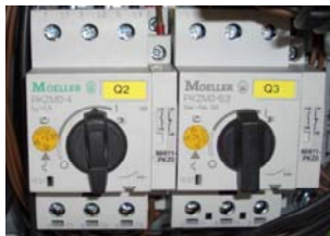
Fig. 1 motor protection switch
